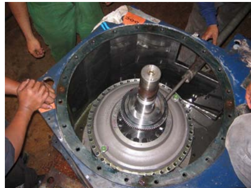
Overhaul Air-Gas Compressor, PTT Sriracha, Boil off compressor
