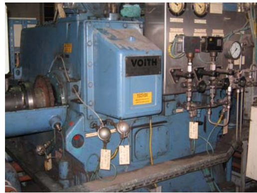
Boiler feed pump and Voith fluid coupling overhaul, 1.2 MW, AA Pulp Mill 2
