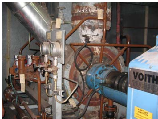
Boiler feed pump and Voith fluid coupling overhaul, 1.2 MW, AA Pulp Mill 2
