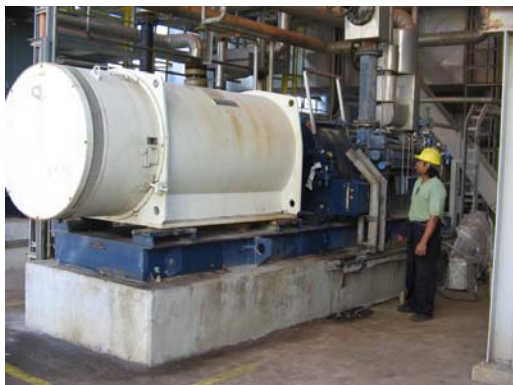
Overhaul Air-Gas Compressor, PTT Sriracha, Boil off compressor
